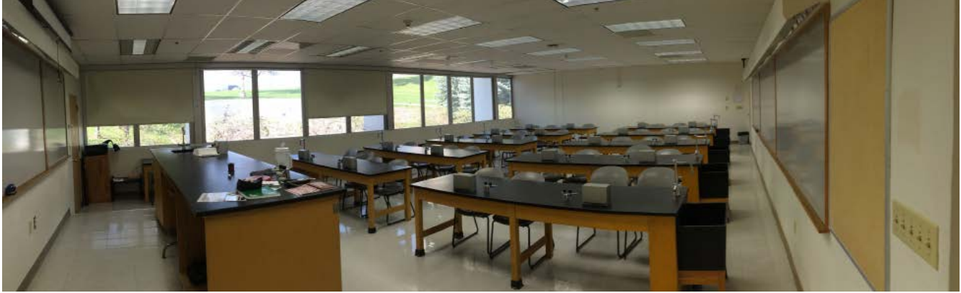
Several classroom spaces have accessibility issues.
